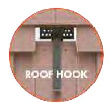
The Roof Hook should NOT rest on the bottom tile. The top tile should sit level with the rest of the tiles.
