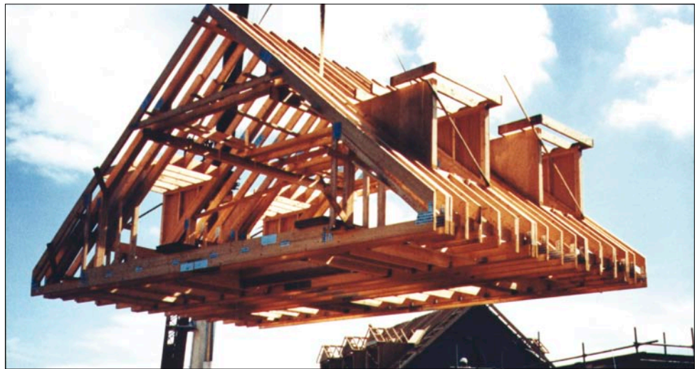
Figure 6 Roof truss built on the ground and lifted into position, avoiding the need to work over open joisting later on
