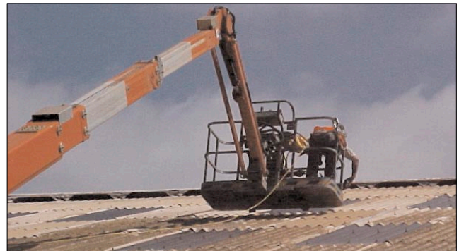
Figure 4 A mobile elevating platform being used to replace a roof sheet
