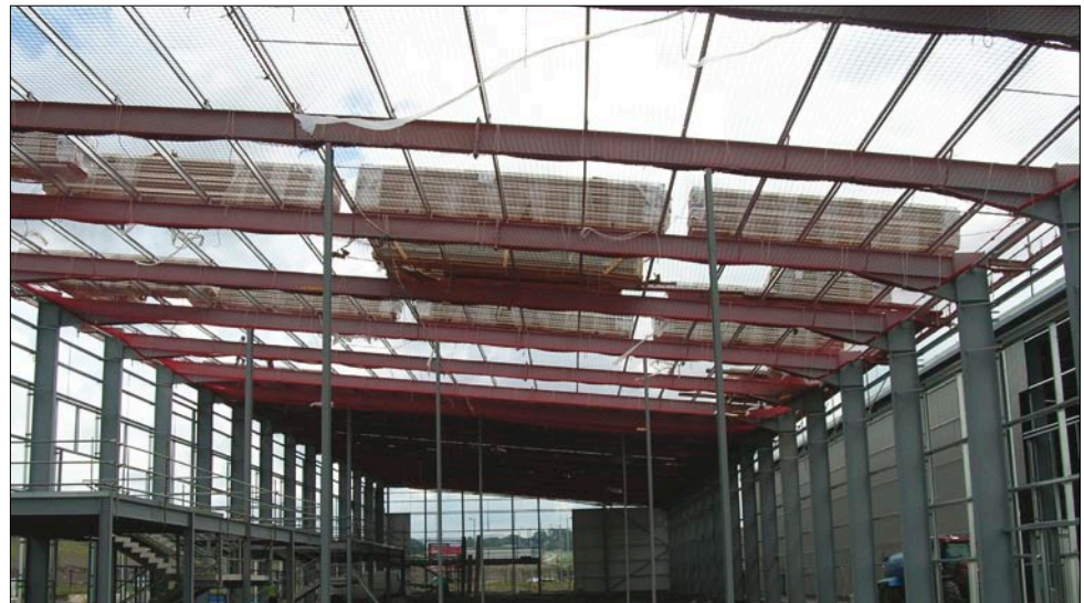
Figure 7 Safety nets installed prior to sheeting. Note that the net is fixed as close to the underside of the roof as possible to minimise the extent of any fall
